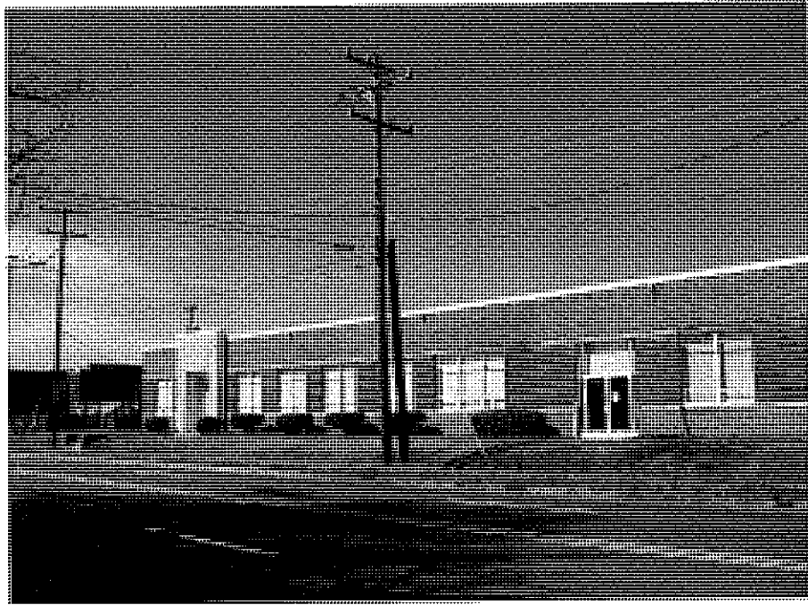
North Graham Street Industrial Historic District (No. 208).
