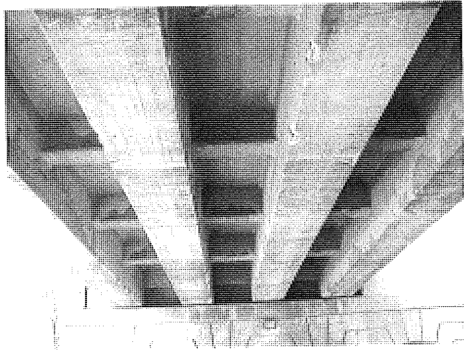
Southern Railway Bridge (No. 210), Substructure.
