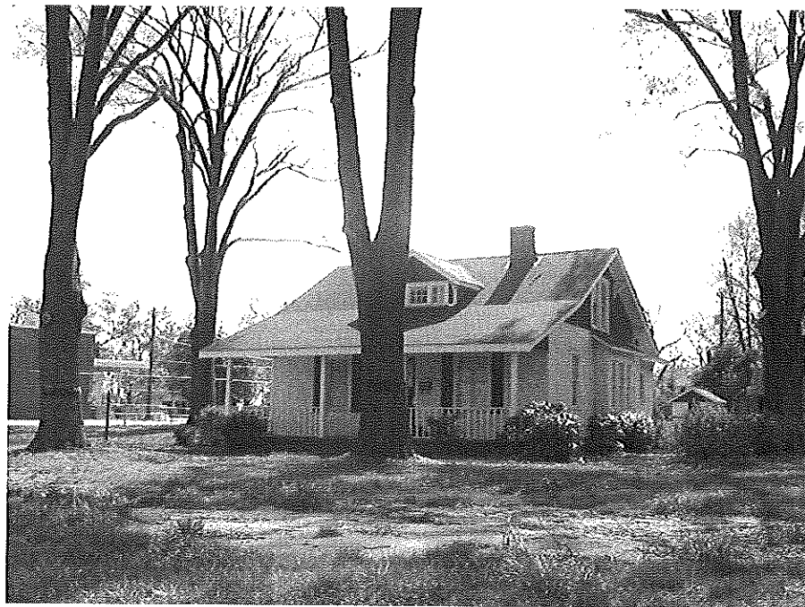
Derita Houses (No. 198).
