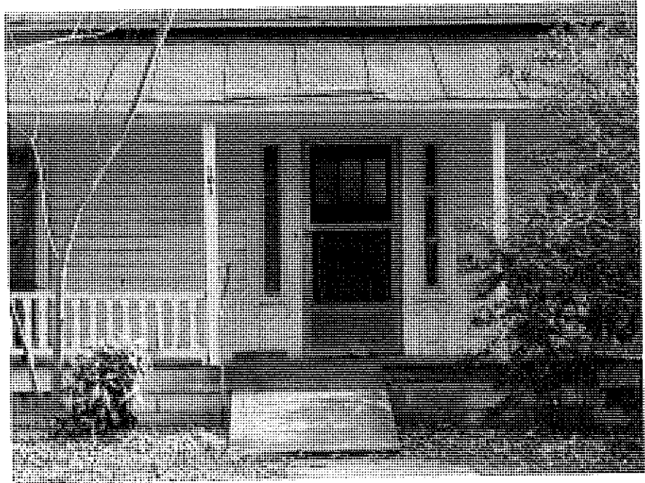
House (No. 159), Entrance.
