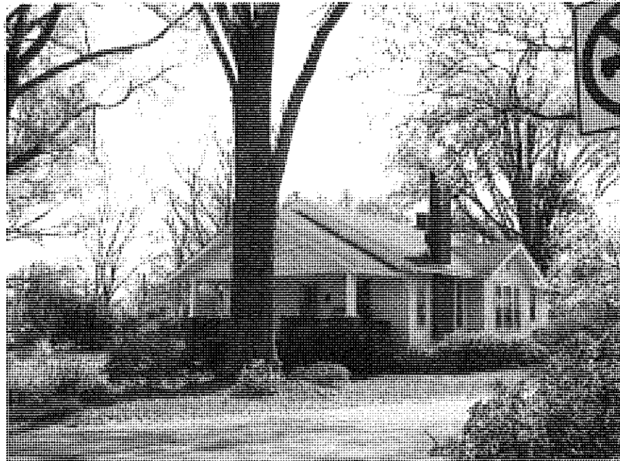
Derita Houses (No. 198).
