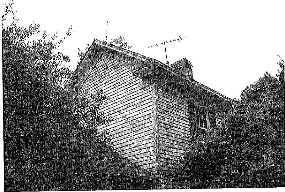
House (No. 79), Cornice and Corner Detail.
