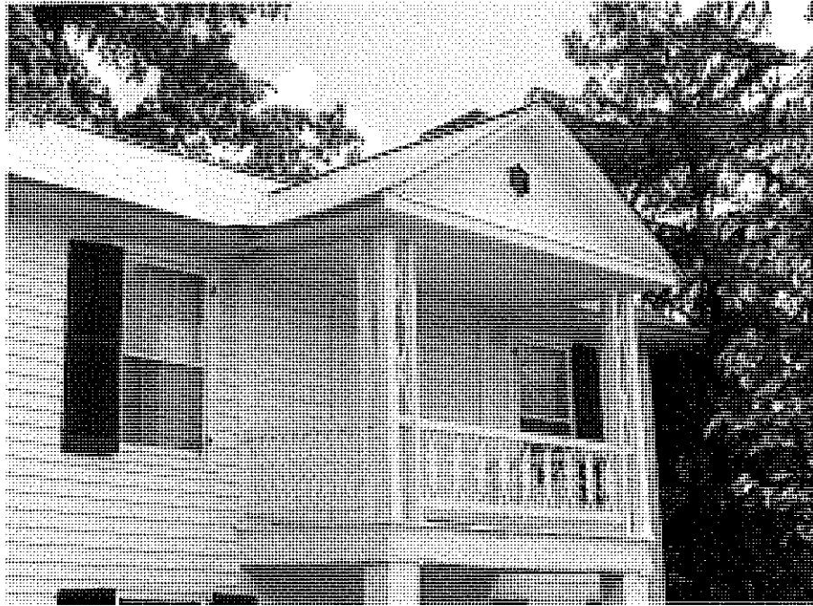
House (No. 82), Porch Detail.
