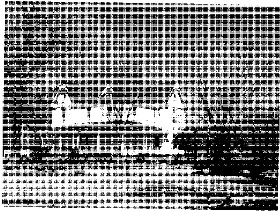
Croft Historic District - Davis House (No. 191).
