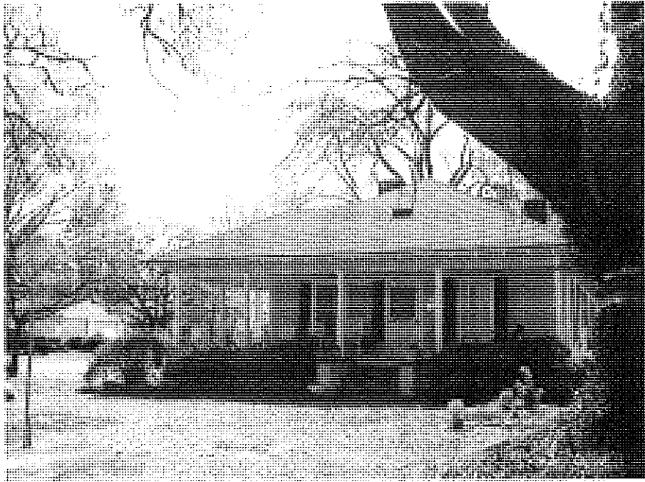
Derita Houses (No. 198).
