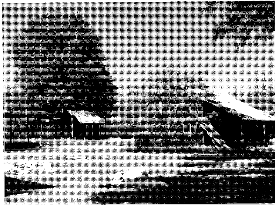
Espy Watt Brawley House (No. 1), Outbuildings.
