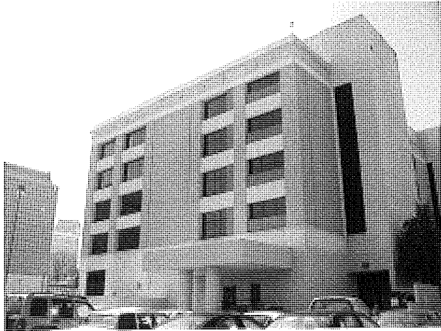
Coddington Building (No. 213), Rear Elevation.
