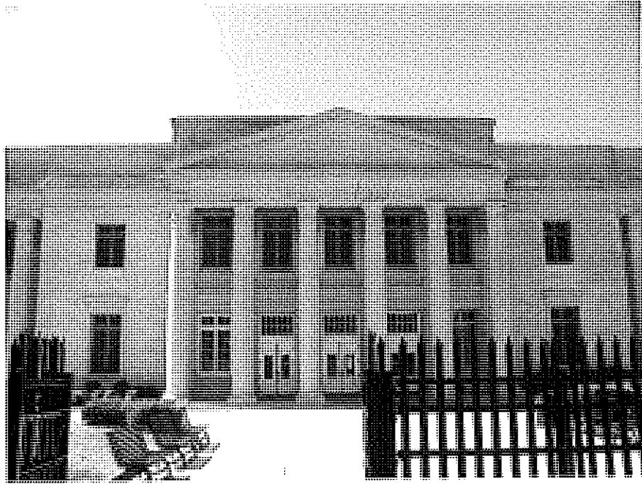
(Former) Charlotte Post Office (No. 216), Front Entrance.
