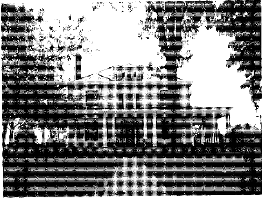
Isaac Harris House (No. 36), House and Setting.
