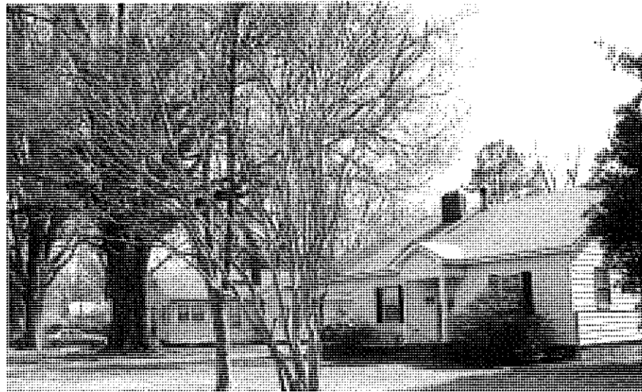
Derita Houses (No. 198).
