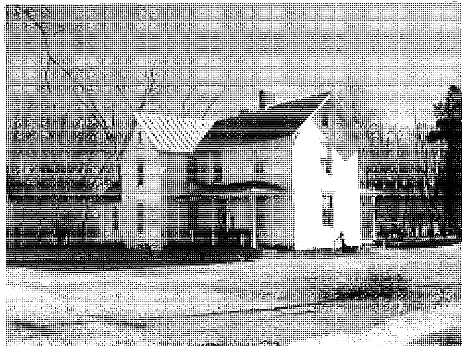
Robbins House (No. 113), House and Setting.
