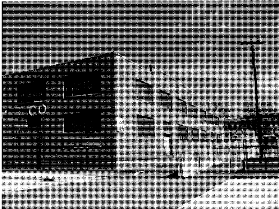
Virginia Paper Company Warehouse (No. 215), Side (East) Elevation.
