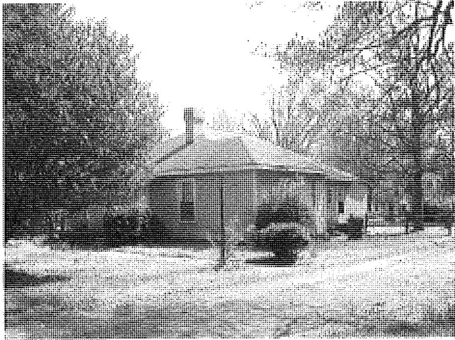
Derita Houses (No. 198).
