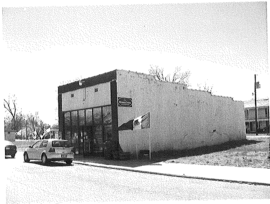
Commercial Building (No. 158).
